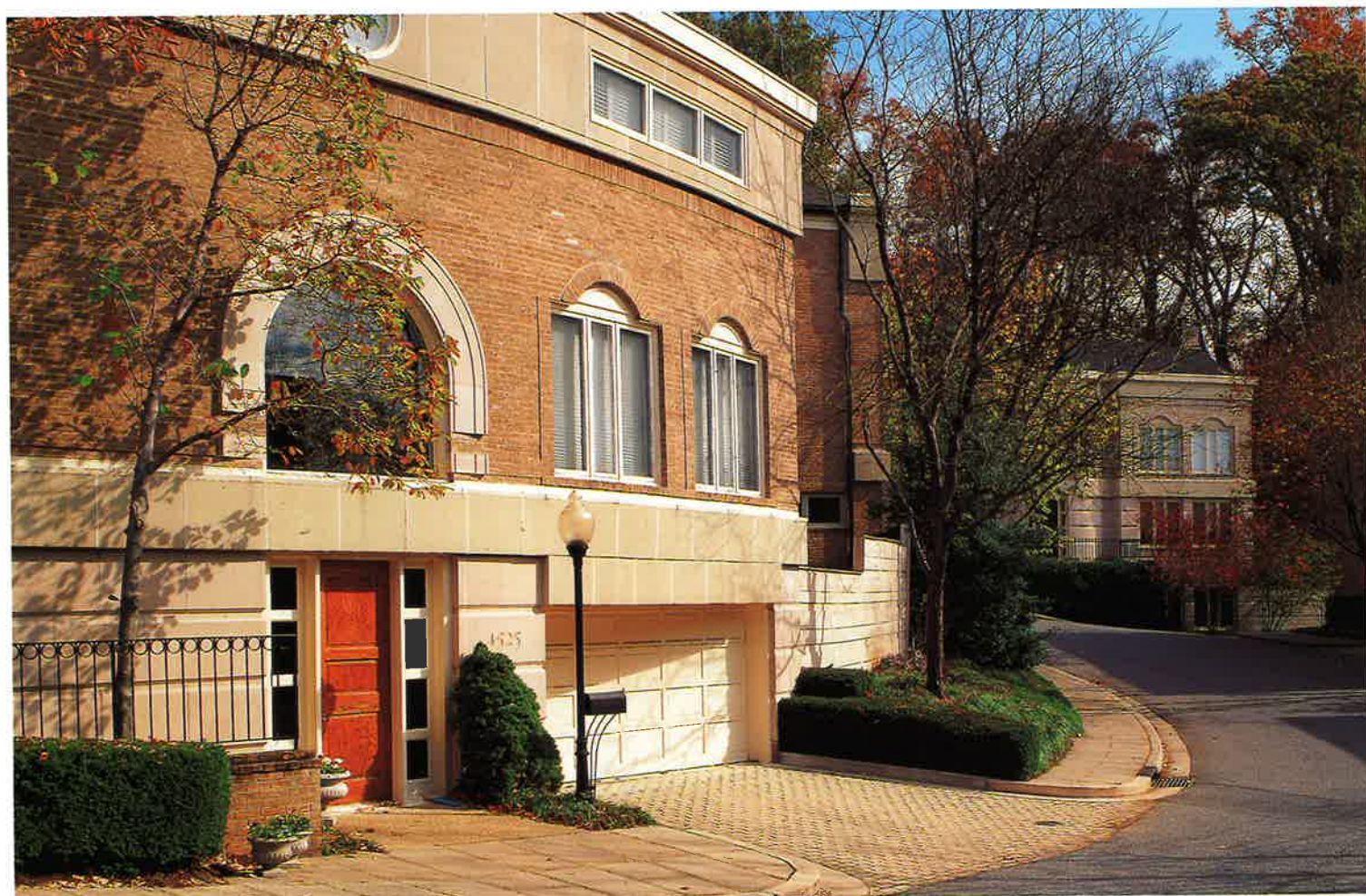
Foxhall Crescents, Washington, DC (Arthur Cotton Moore Associates)
