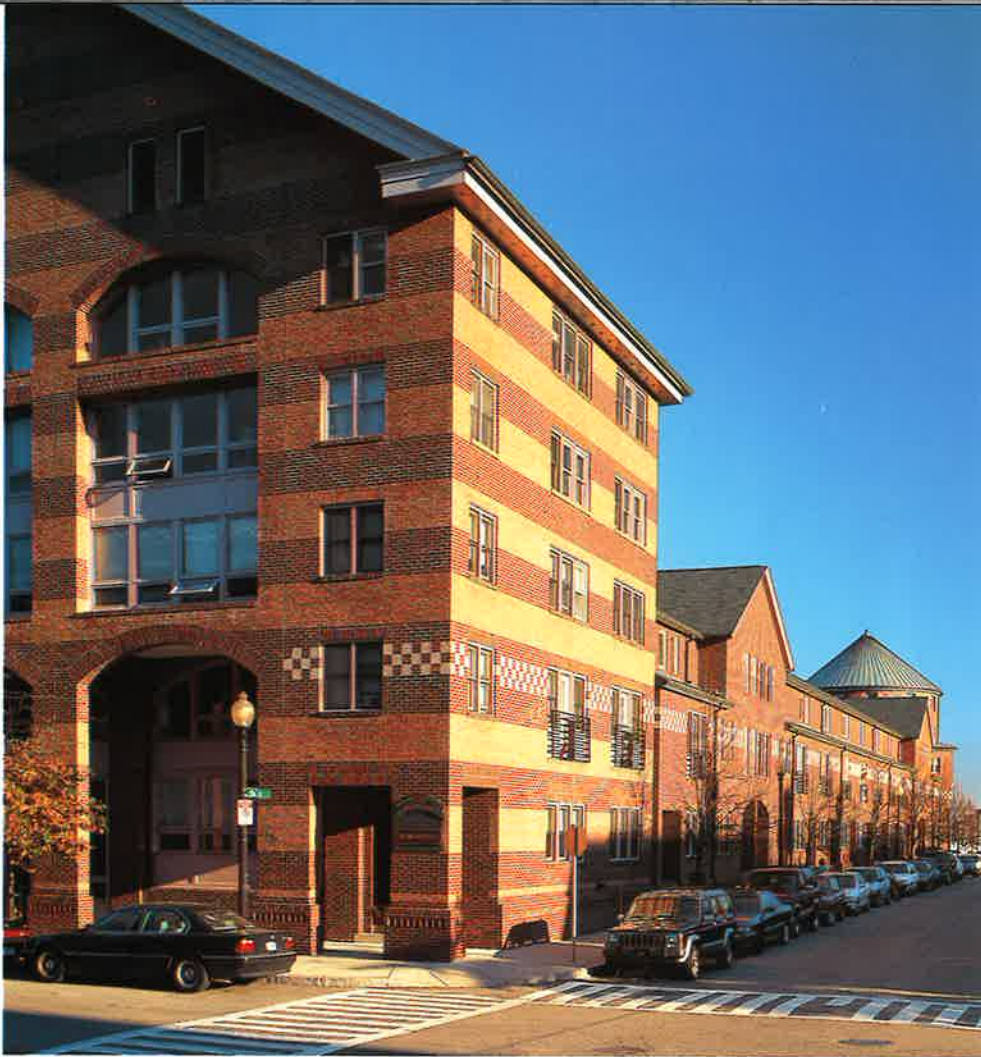
Charlestown Navy Yard Rowhouses, Boston (William Rawn Associates)
