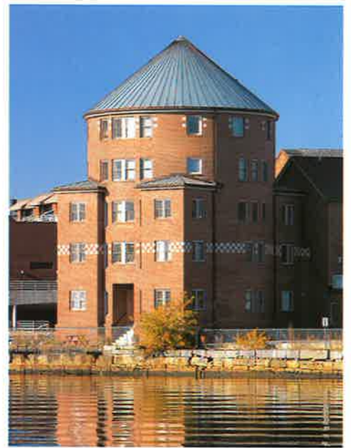
Charlestown Navy Yard Rowhouses, Boston (William Rawn Associates)
